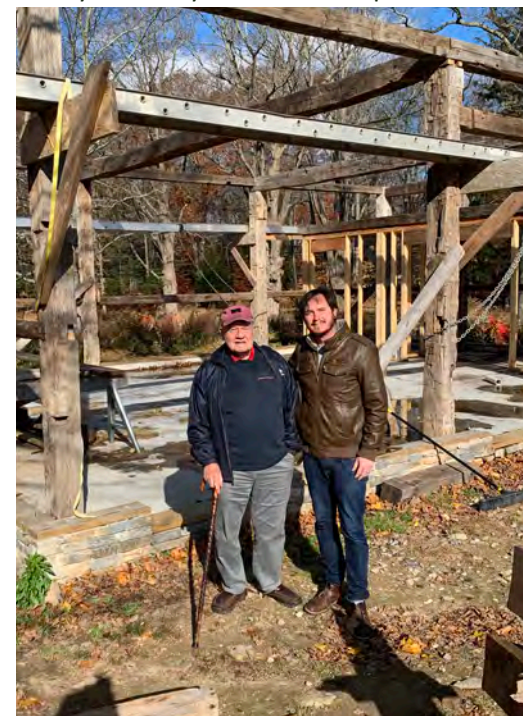
Robert Russell with David McCarthy, Executive Director, standing in front of the under-construction Daniel Offutt Barn at Chestnut Meadows
